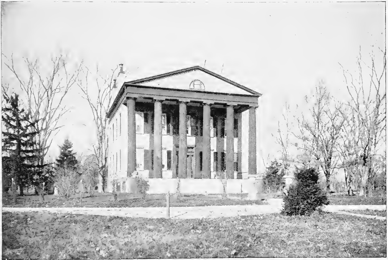
WOODBURN HALL THE CHRISTOPHER B. MILLER HOMESTEAD—New Windsor
